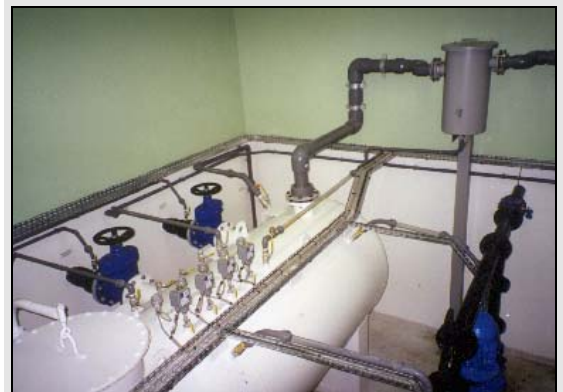
Vacuum vessel and associated equipment
