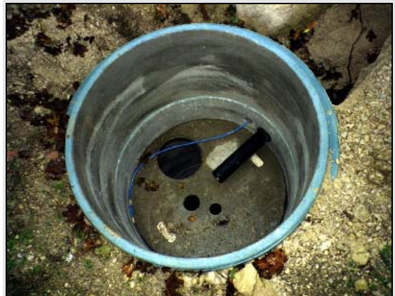
Valve chamber installed
